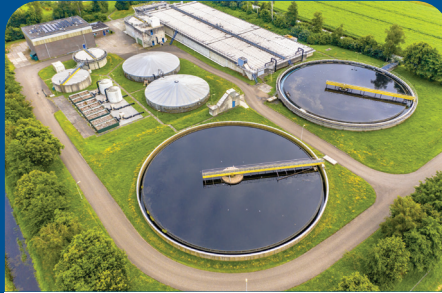
Water & waste water treatment plants
