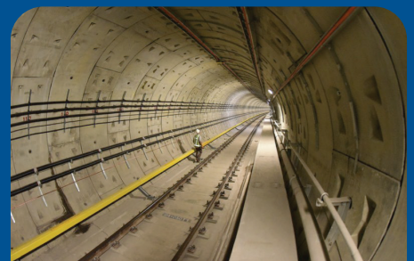
Tunneling & temporary reinforcement
